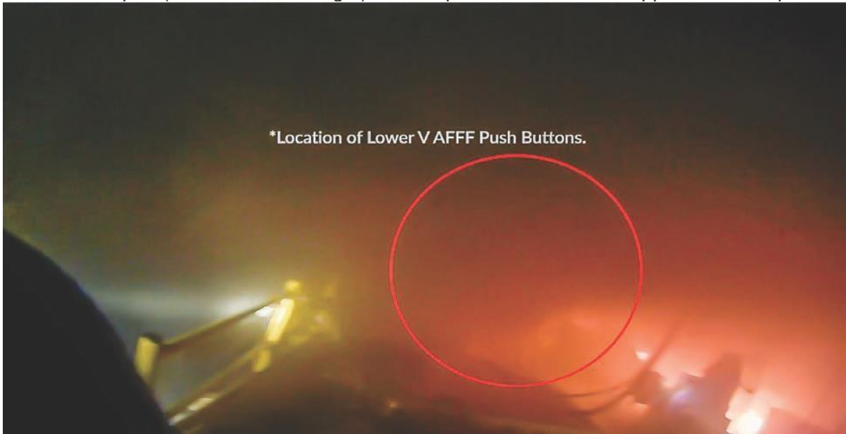
81 Figure 33, Still photo captured from GoPro video provided by San Diego Fire Department (SDFD) showing the location of AFFF push-buttons on 12 July 2020 after SDFD made entry into the vehicle stowage area via the sideport.
